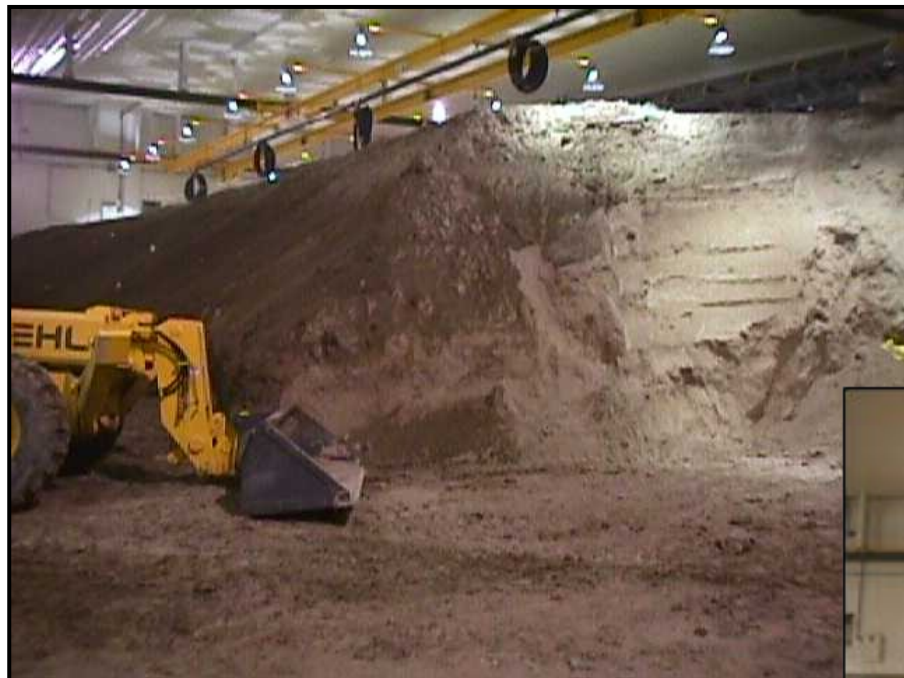
Soil berm inside of TSA-RE during initial soil removal
