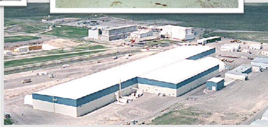
Large Butler Building built over soil covered berm, 1996
